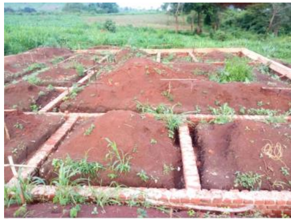
Photo 12. Ongoing construction at Kikonga primary school, Kisanga village in Kilosa
