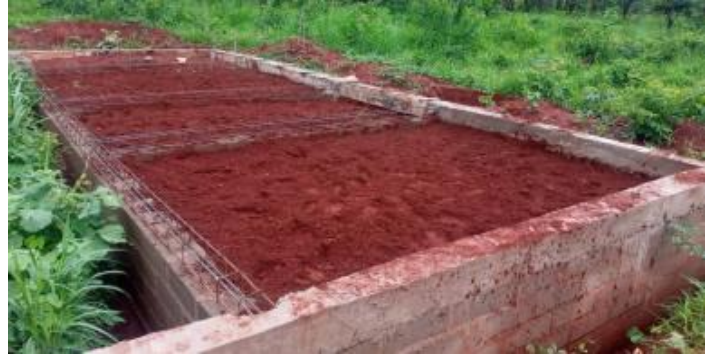
Photo 10. Ongoing construction of Kitunduweta village dispensary in Kilosa
