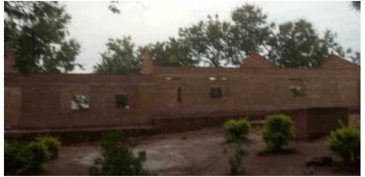
Photo 8. Ongoing construction of 3 classrooms at Nyali village in Kilosa.
