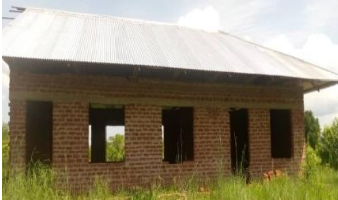
Photo 9. Ongoing construction of Mahara primary school classroom in Mvomero
